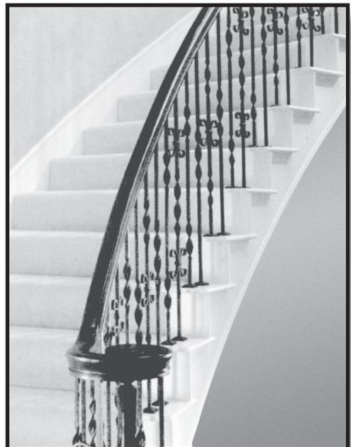
Installation combining Ribbon and Butterfly Iron Balusters and M022 shoes with Oak Handrail, Volutes and Newels
